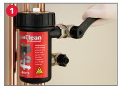
IMPORTANT – Before commencing any servicing work, turn off electrical supply to the boiler. Ensure the water is not too hot to undertake work on the system. Turn off both isolation valves to the marked OFF position. Loosen the air vent to release internal pressure. When venting, protect the surface beneath the MagnaClean Professional with a dust sheet or container to capture any drops of water.
