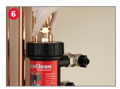
Open the isolation valves to the marked ON position and vent/bleed through the Pro-Fill air vent. Protect the surface beneath the MagnaClean Professional with a dust sheet or container to capture any drops of water. Run the central heating system while checking for leaks. Repeat servicing steps 1 - 6 if required. Ensure the filter is thoroughly clean before leaving the premises.
