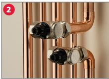
Using a suitable cutter, carefully remove the marked section of pipework to create the correct opening. Prepare the pipe and fittings accordingly. Lubricate the olives and assemble the valves on the pipe.
