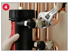
Loosely secure the MagnaClean Professional to the valves. Grip the MagnaClean canister and tighten the compression fittings being careful not to over tighten.
